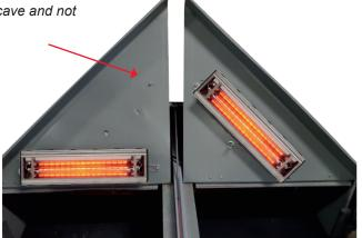
UniHeater is mounted with brackets facing the cave as well. There is an angle on the dish inside UniHeater, this provides a better dispersion of heat in the cave. When you installed correctly.
